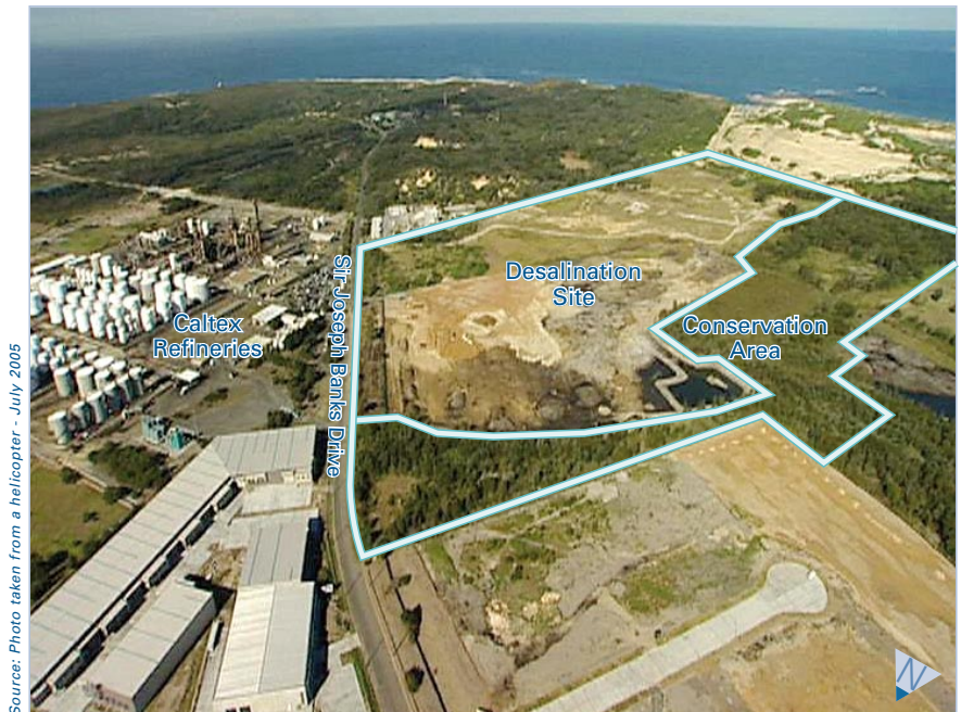
Figure 4.2 Desalination plant site
